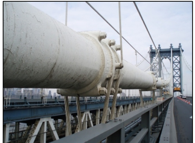
A cable on the Manhattan Bridge
